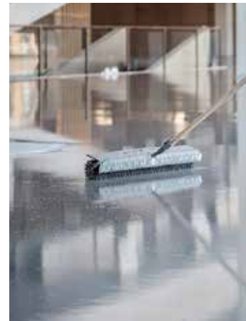
6. Apply UZIN NC 195 with a thickness of approximately 8 mm
