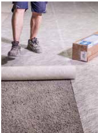
4. Installation of the renovation fleece UZIN RR 201 with 2 cm overlap
