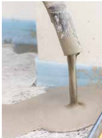
5. Application of thin screed UZIN NC 195
