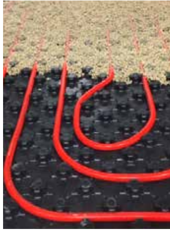
2. Backfilling of the space between the nubs with SYMPOR-LB 400 (or Sympor LB 400 S)
